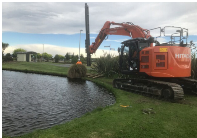
Driving the first pile
