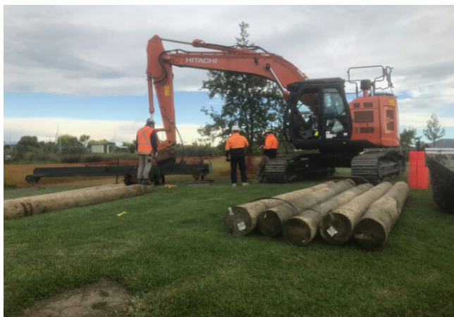
Bridge piles assembled
