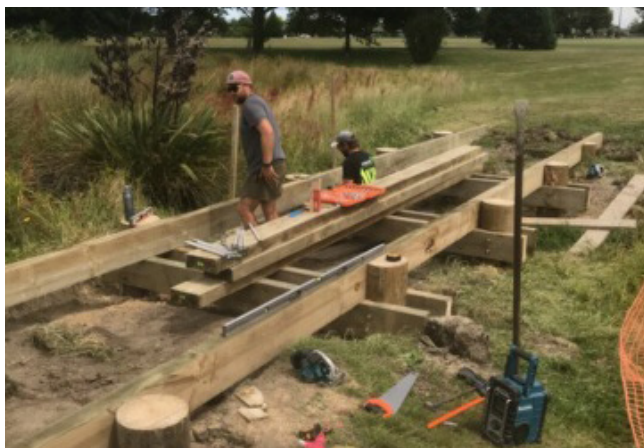
Cross beams & bearers added
