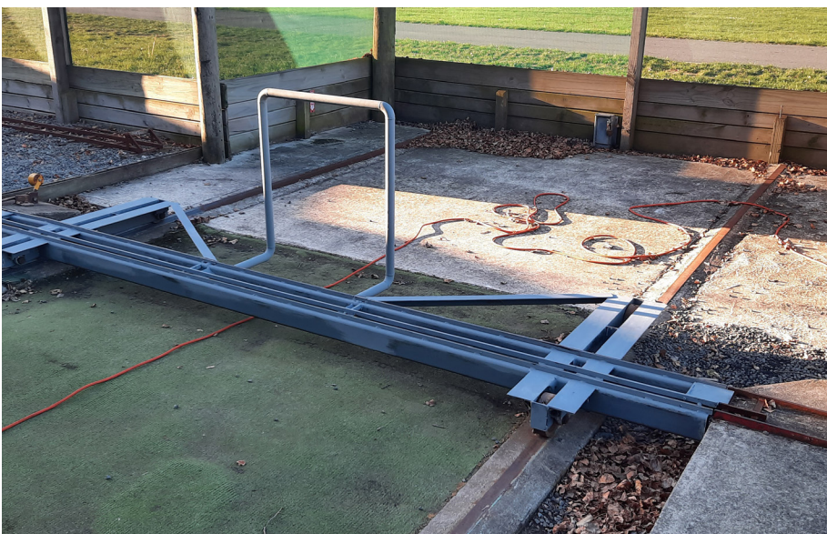
New traverser: Paint job by Keith Robson
