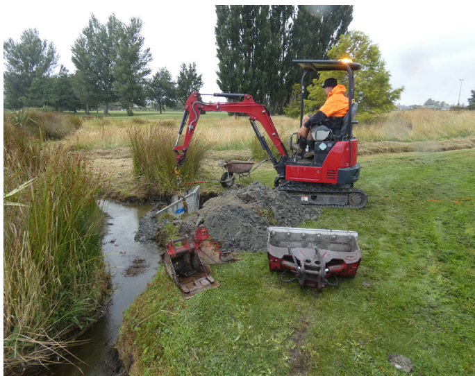
Placing pre-cast form into position
