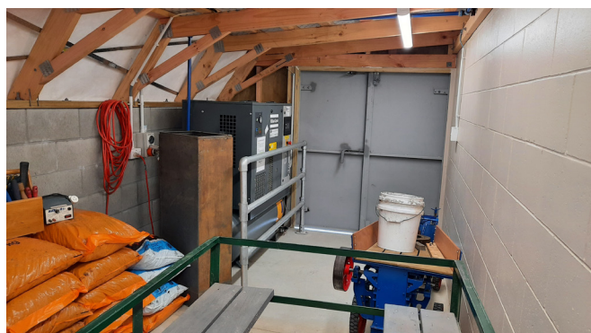
Inside the new loco shed extension. New air-compressor nearest the l.h. door.
