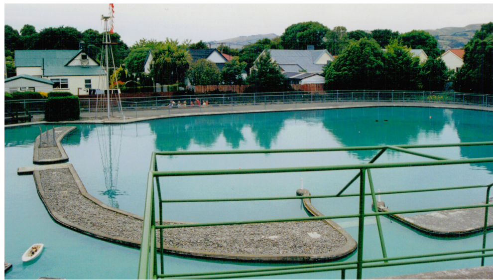
Pond (note safety fence to prevent railway passengers from falling in)
