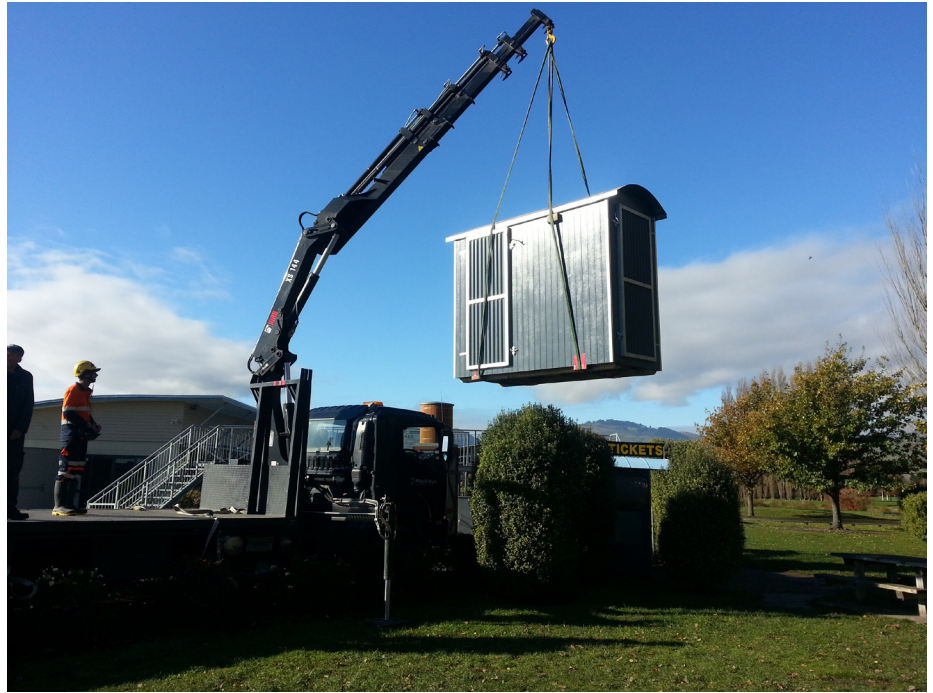
Hoisted into position
