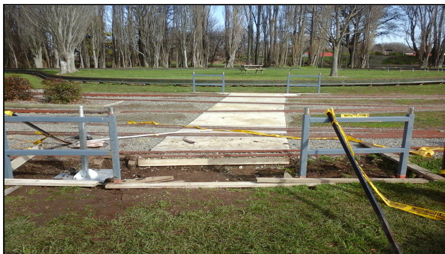
The new crossing nears completion
