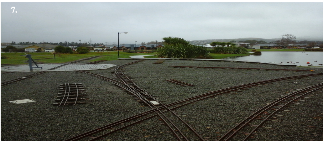
7. The new "park-up" track
